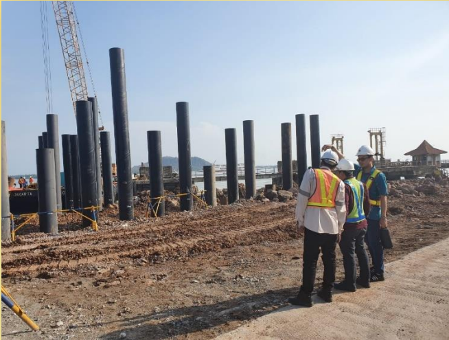
Construction and Piling work for Dock IV Merak – Bakauheni ferry ports
