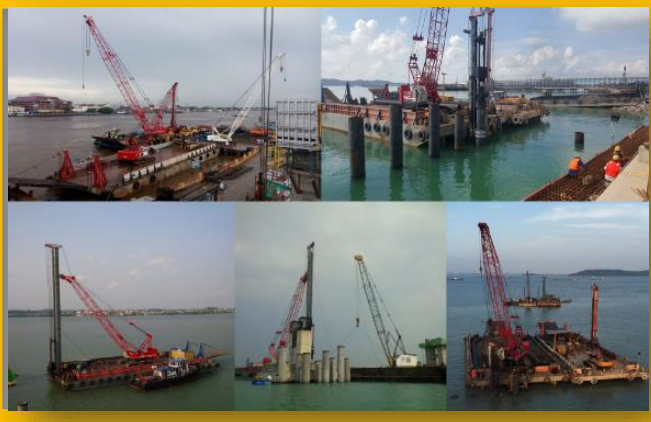
Foundation & Retaining Wall
