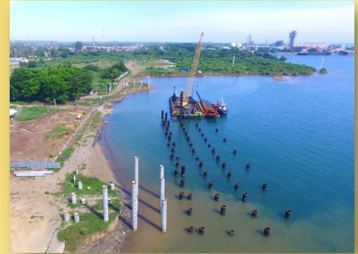
Piling Work for Offshore Project NPK Chemical Plant Kap 500,000 Mtpy Pim
