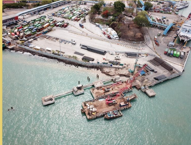
Bored Pile & Piling for Construction Project of Dock IV Merak – Bakauheni
